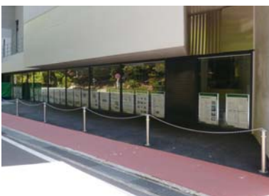
Isolation Structure Gallery
