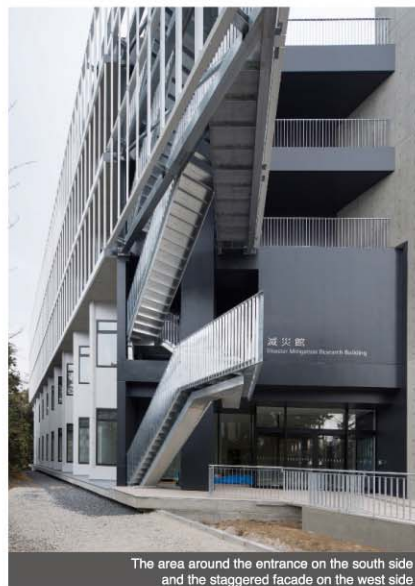
Appearance of the south-west side
